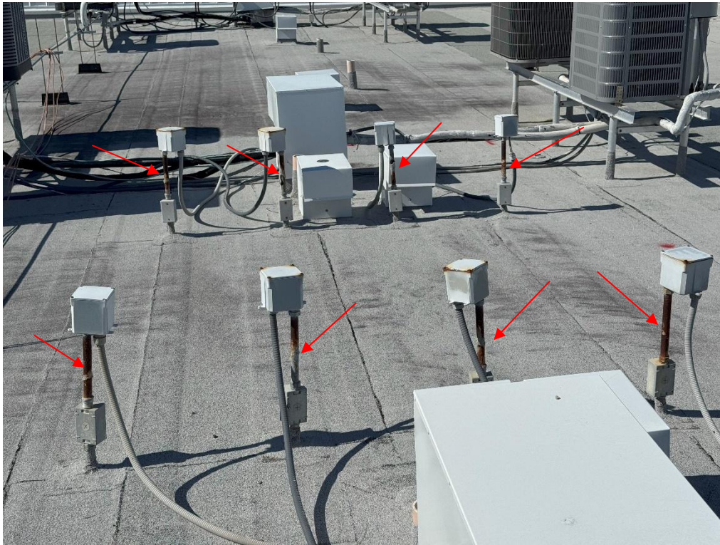
Photo 13: Rusted electrical conduit on the roof
