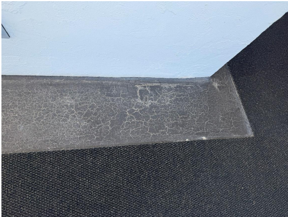
Photo 14: Typical failing coating along elevated walkway slabs
