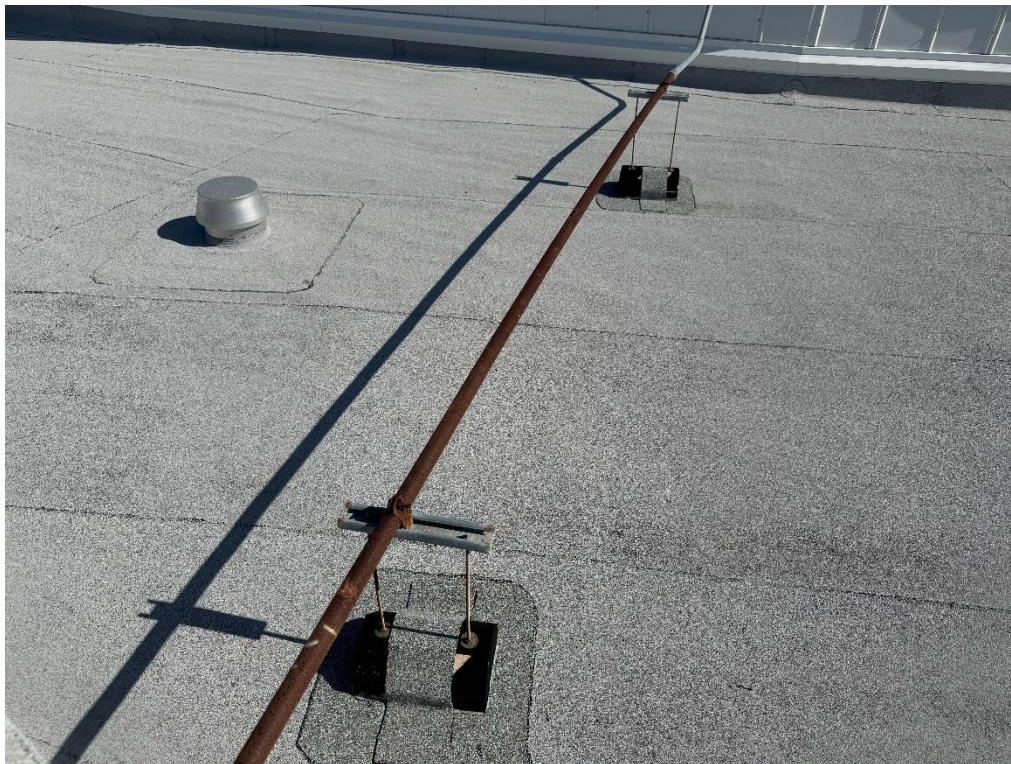
Photo 12: Rusty electrical conduit on the roof
