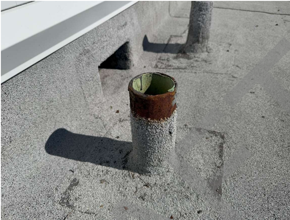
Photo 7: Ventilation Pipe with lining
