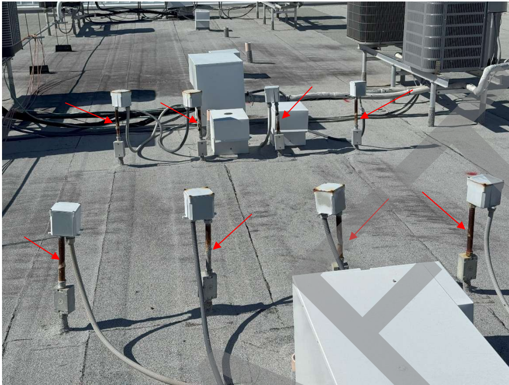
Photo 13: Rusted electrical conduit on the roof
