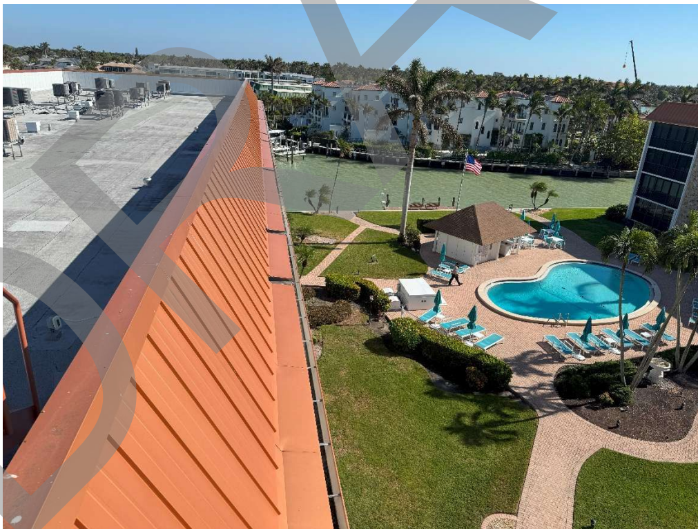
Photo 4: General condition of standing seam metal mansard roofs
