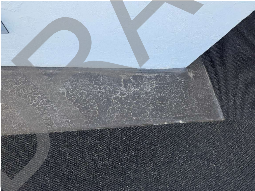
Photo 14: Typical failing coating along elevated walkway slabs
