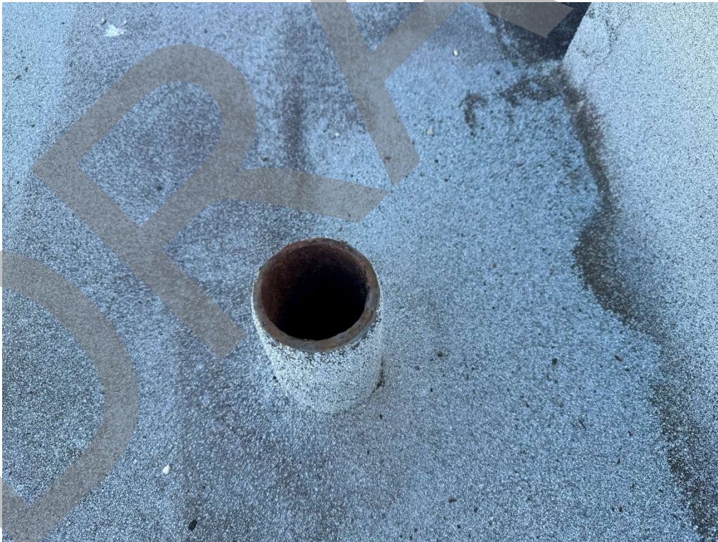
Photo 8: Ventilation Pipe without lining
