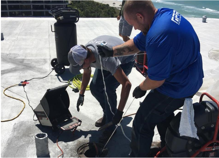
PULL LINER INTO PLACE
