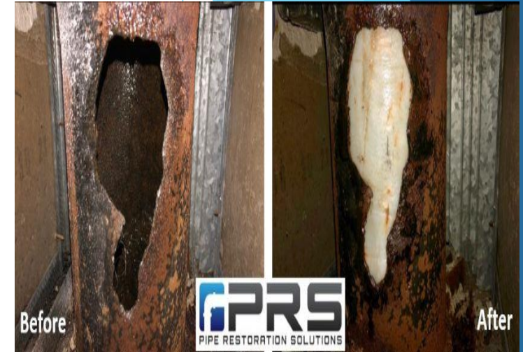
FINAL POST-LINING INSPECTION
