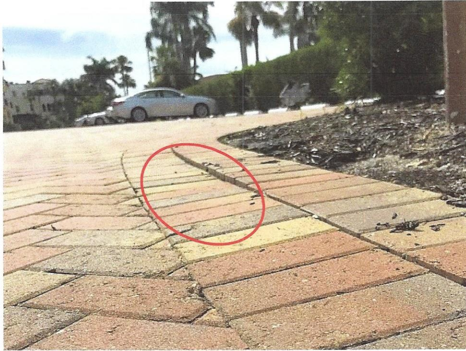
Photograph 19: Localized area of depressed pavers at the southernmost entrance to the community
