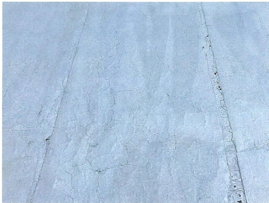
Photograph 4: Cracking throughout the liquid membrane and cap sheet on the West Building Roof
