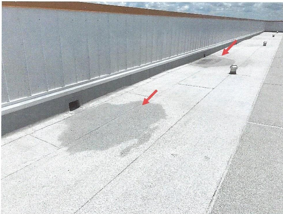
Photograph 2: Standing water near scuppers on the north side of the North Building Roof
