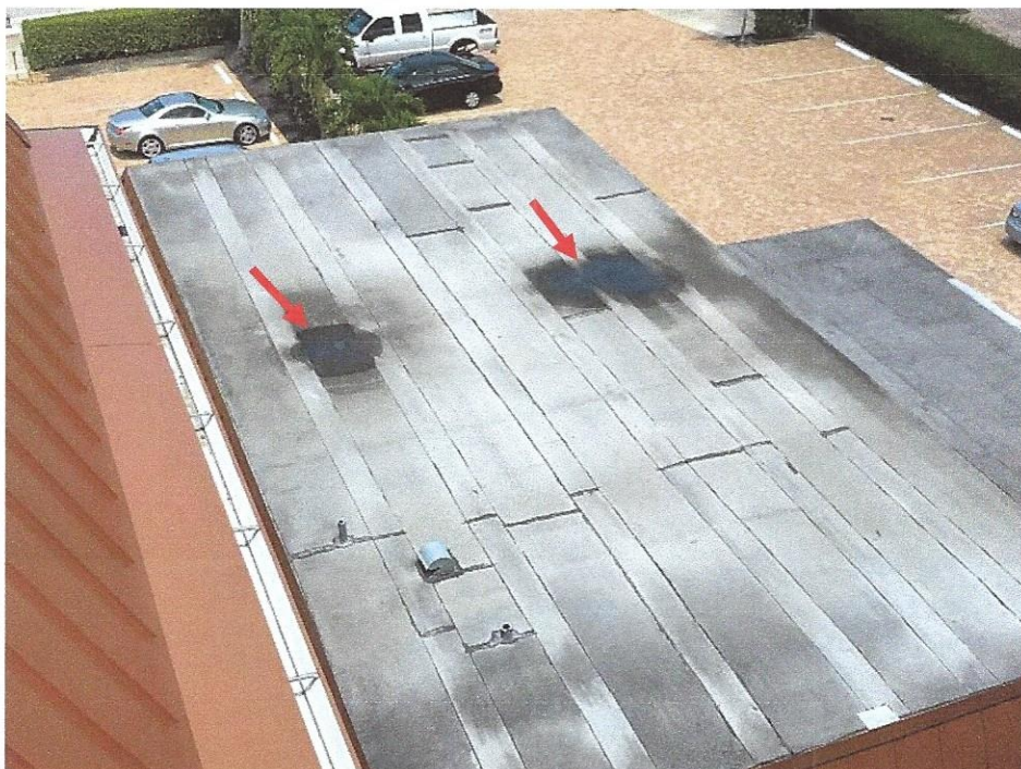
Photograph 6: Office Building Roof and areas of standing water
