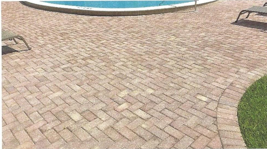
Photograph 25: Typical Pool Deck and Walkway Pavers
