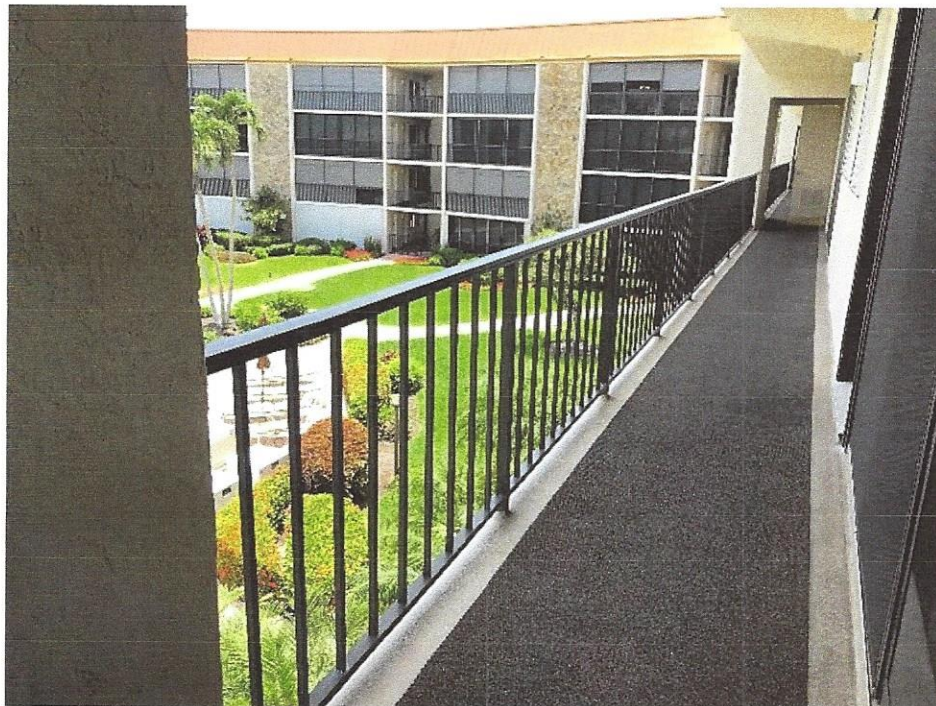
Photograph 12: Typical Aluminum Walkway Railings
