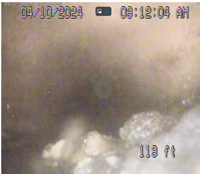
Main Line with sand and major build up
