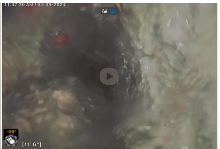
From unit 107 to unit 108 major ledging and build up
